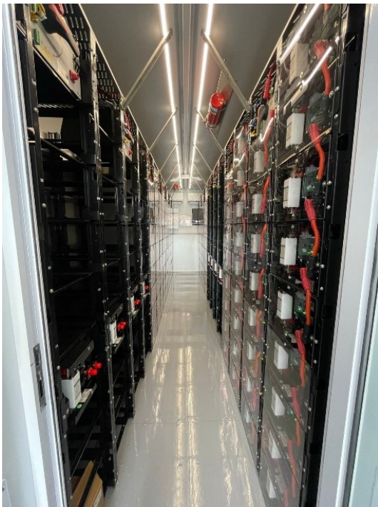
Emergency battery energy storage system (BESS)
