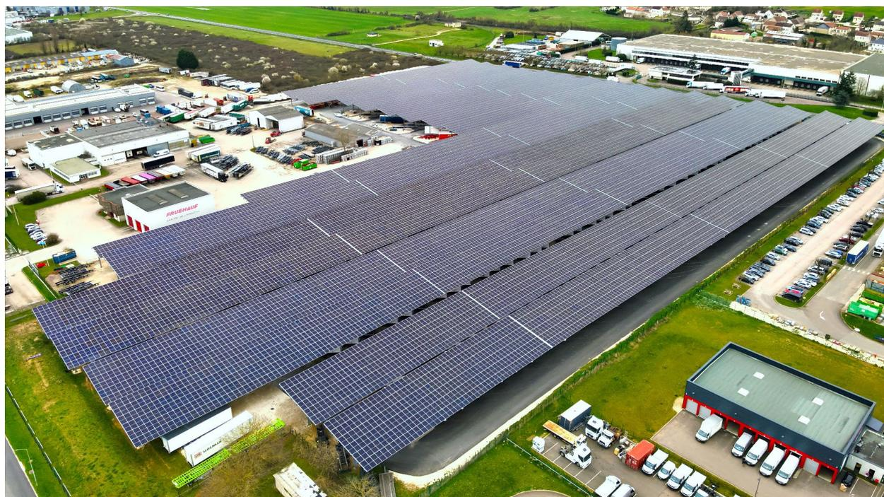
The Fruehauf production site in Auxerre, employing 650 people, will now be equipped with **16 photovoltaic carports** with a **height of more than 5 metres**, covering an area of **52,000 m<sup>2</sup>**. These carports, whose **lengths vary between 150 and 350 meters**, will make it possible to install a **total capacity of 11 MWp**, generating an **estimated annual production of 12.7 GWh**, equivalent to the energy consumption of **2,800 inhabitants**.
