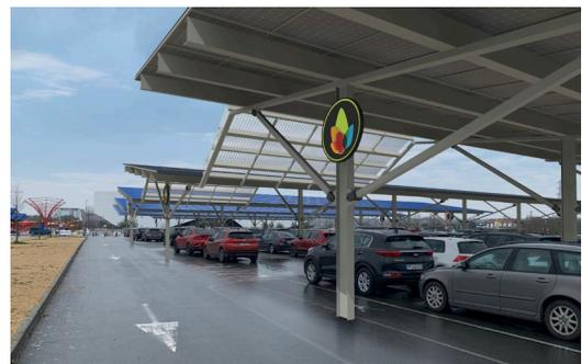
Walibi Rhône-Alpes will benefit from **5.6 MWp of solar carports (a mix of self-consumption and grid injection)** with an **annual production of 6.5 GWh** and will offer **30 charging points for electric vehicles**. Construction, which also began in January, is expected to be completed by December 2025.
